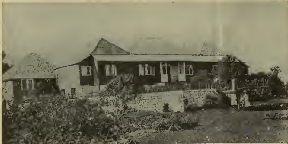
Typical planter's house. The three roofs are a protective device against high winds
